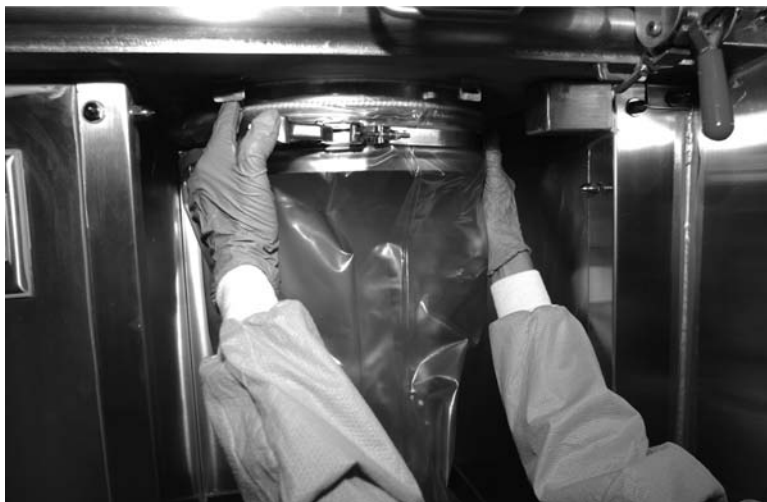
Figure 17.4 A typical bag-out port.
